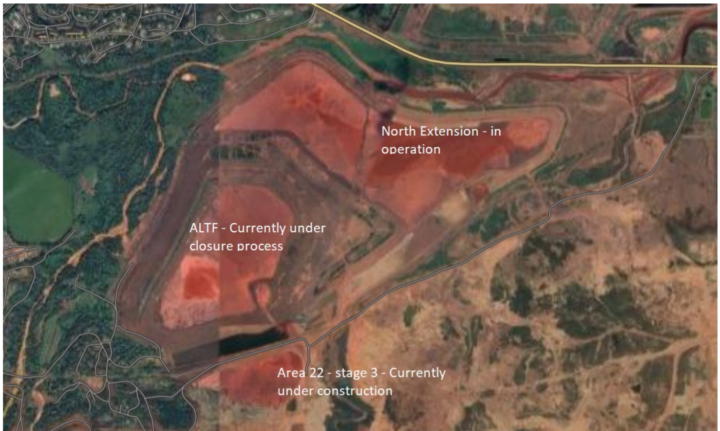
Figure 2: Tailings Management Facilities
