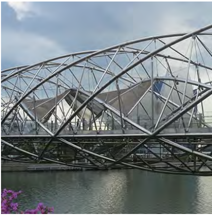
PICTURED HERE IS THE HELIX BRIDGE IN SINGAPORE, MADE FROM NICKEL-CONTAINING STAINLESS STEEL. THE CORROSION-RESISTANT PROPERTIES OF STAINLESS STEEL ARE EXCELLENT FOR THE HUMID CLIMATE.
