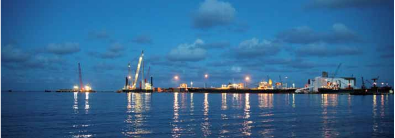
New bulk port facility at Toamasina, Madagascar
