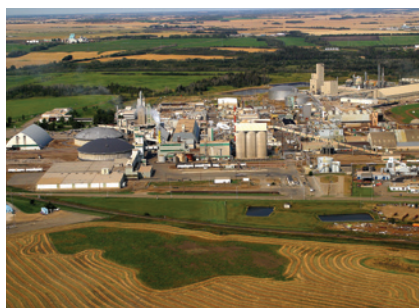
The Fort Saskatchewan refinery site has been operated by Sherritt companies since 1954.
